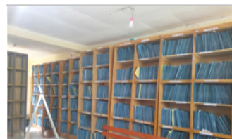
MRU Renovation & Shelving
