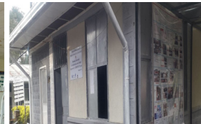
After Renovation MRU
